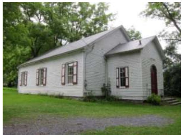
Fig.12. The former Presbyterian Church in Allen Township 18 which served the large Scots-Irish community but also held Reform Church services. This is the third building on the site and was built in 1813 19 after Simon Jr. died. Photo by M. Falconer 2010.
