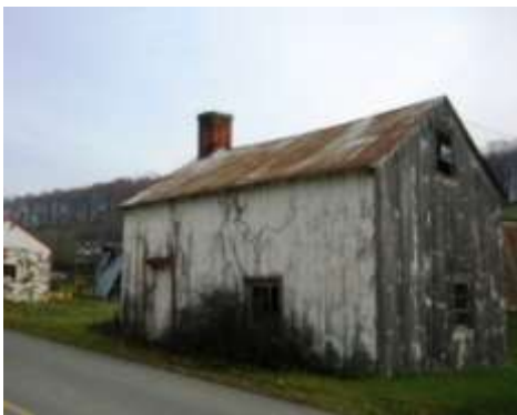
Fig. 1. This 200 year old log cabin is similar to the kind of small log house that Gucker would have built. The exterior of even this small house was weather boarded with vertical boards. Photo by M. Falconer 2010.
