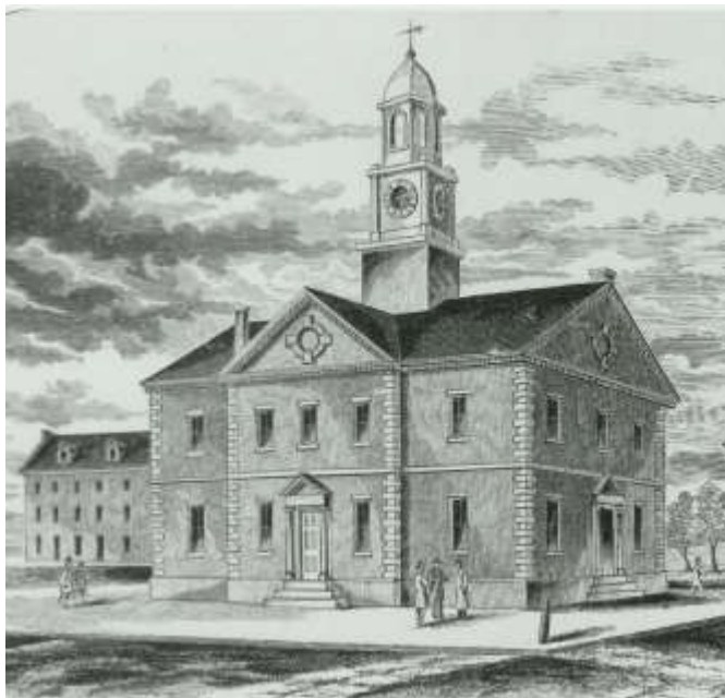
Fig. 18. The old court house in Lancaster – the place where the Pennsylvania General Assembly met after fleeing Philadelphia.
