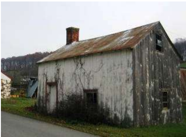
Log cabin on what was Jost Dreisbach's property. Exterior is covered by boards. Probably built about 1790.
